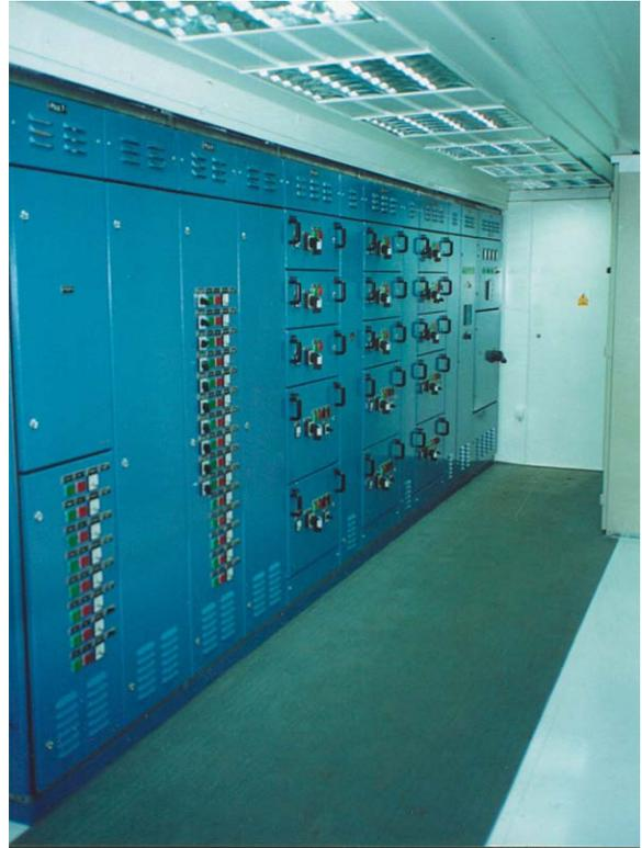
*Front side view of the draw-out type panel-switchgear 400/231V for technological consumers. High wattage consumers are located in drawers (middle part of the switchgear) and low wattage consumers - on montage plates (left side of the photo)*
