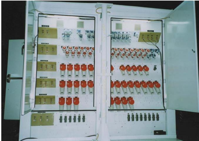
*Board with plug-in sockets for connecting external consumers.*
