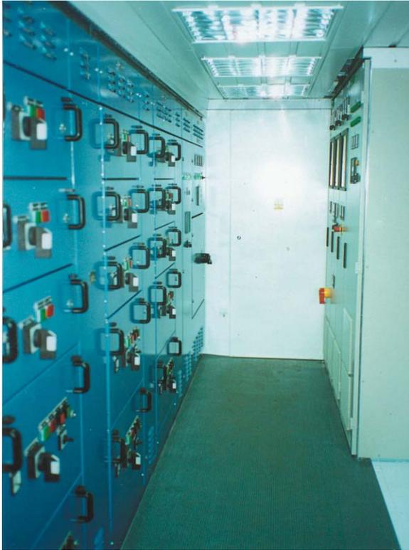
*View of the draw-out type panel-switchgear 400/231V for technological consumers of power 75kW together with the 6-stage capacitor battery 275kVar (left side of the photo). To the right there is the panel switchgear 690V for 6 motors with inverters and 3 capacitor batteries 600kVar.*
